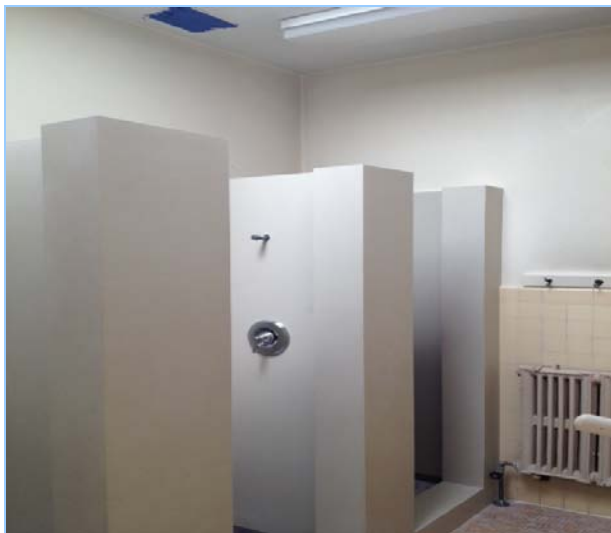
Fire Station #6 New Showers
