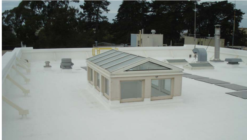
Fire Station #40 New Roof
