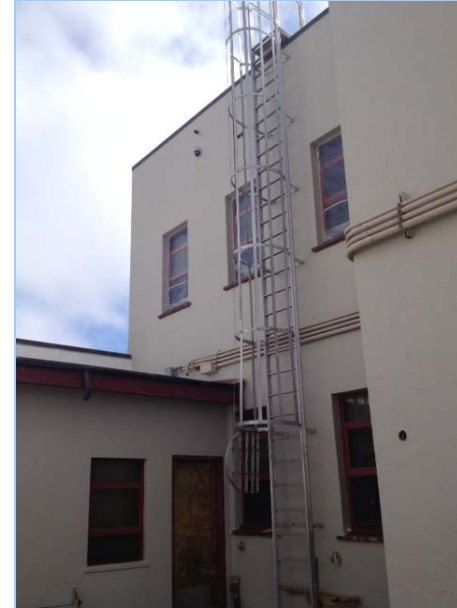
Fire Station #40 Paint - after
