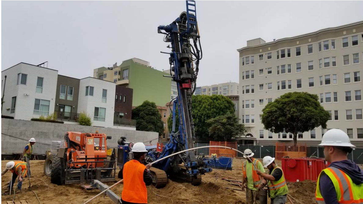
Fire Station 5 – Drilling and Placement of Soil Micropiles (August 15, 2017)
