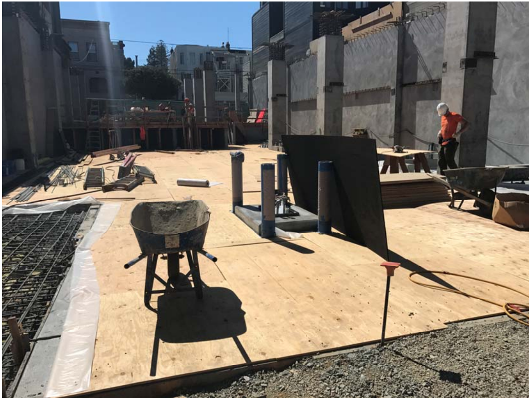
Fire Station 16 – 1st Floor Lower Level Concrete Slab (September 25, 2017)
