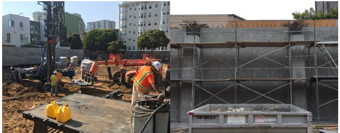
FS 5 Drilling and Placement of Micropiles
