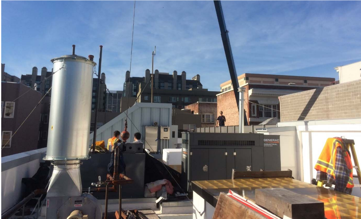
FS 3 Roofing, HVAC, and Generator Replacement
