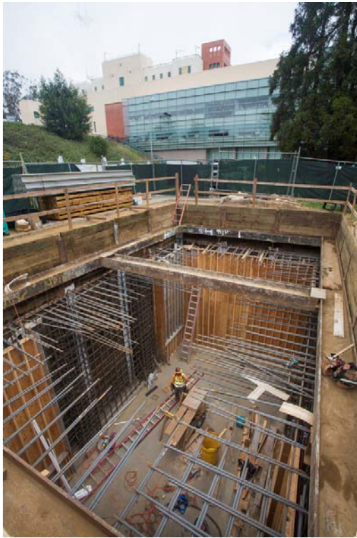
Laguna Honda Hospital cistern
