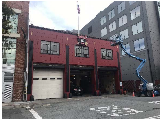
FS 8 – Exterior Envelope – In Progress
