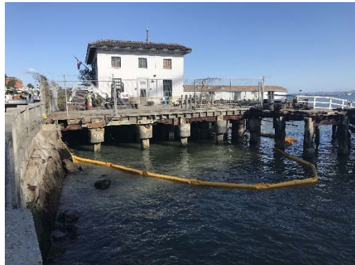
FS 35 – Pier 22 1/2 Demolition (September 30, 2019)
