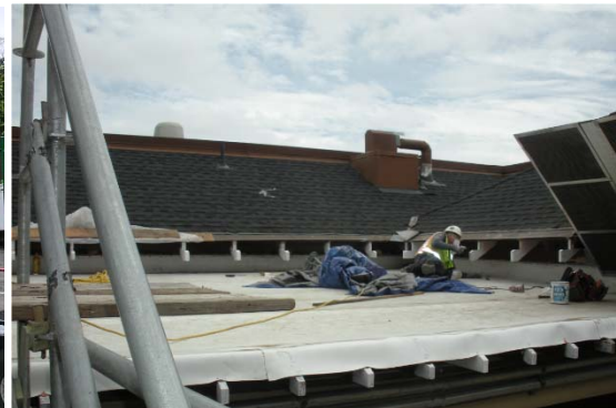
Rafter tail replacement.
