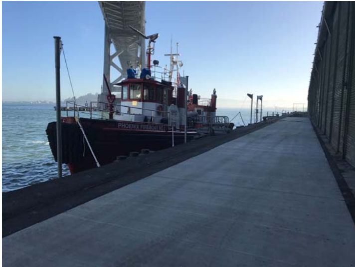
Pier 26 Fireboat Berths – Phoenix Fireboat Moored at Pier 26 (March 28, 2018)
