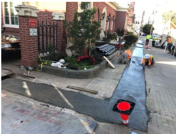
Richmond Station – trench, install storm pipes, backfill and re-pave road.
