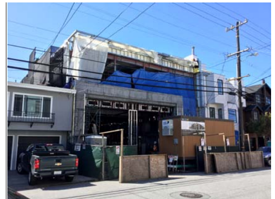
Fire Station 16 NE View from Greenwich Street
