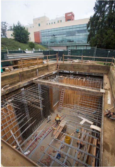
Laguna Honda Hospital cistern
