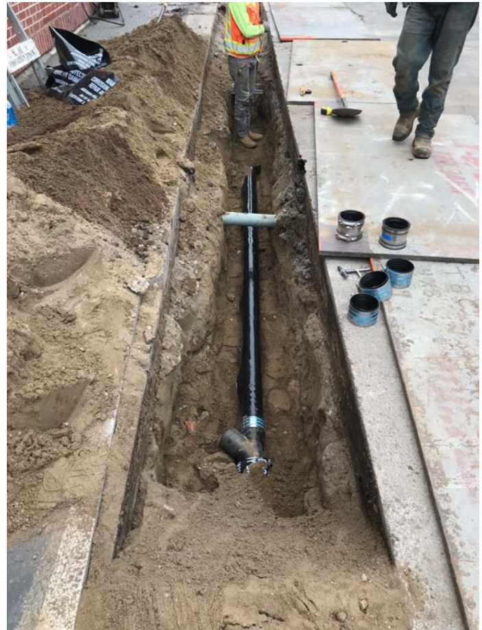
Richmond Station – trench, install storm pipes, backfill and re-pave road.
