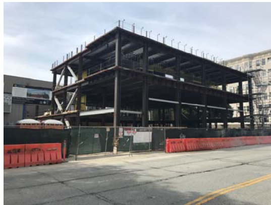
Fire Station 5 SE View from Webster Street
