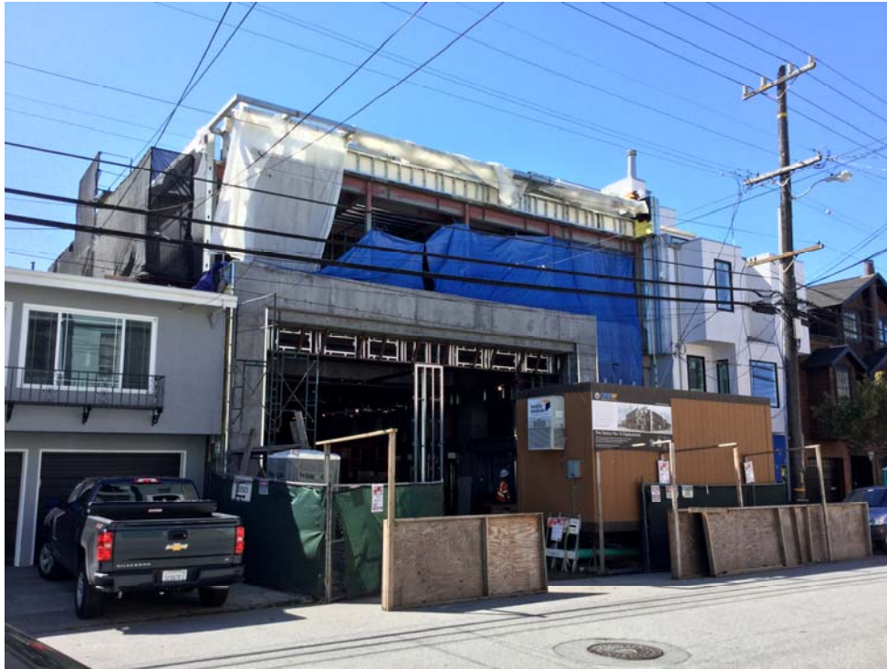
Fire Station 16 – View of North Elevation from Greenwich Street (3.26.18)
