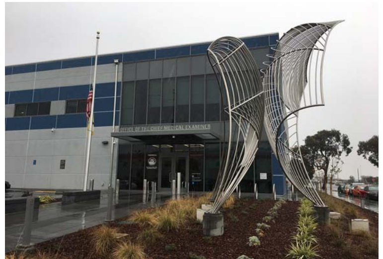
OCME SE Building View from Jennings Street
