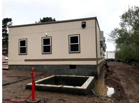
Building – side view
