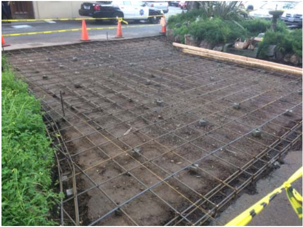
Park Police Station – Left: existing asphalt pavement being demolished, rebars installed. Right: new accessible parking space.
