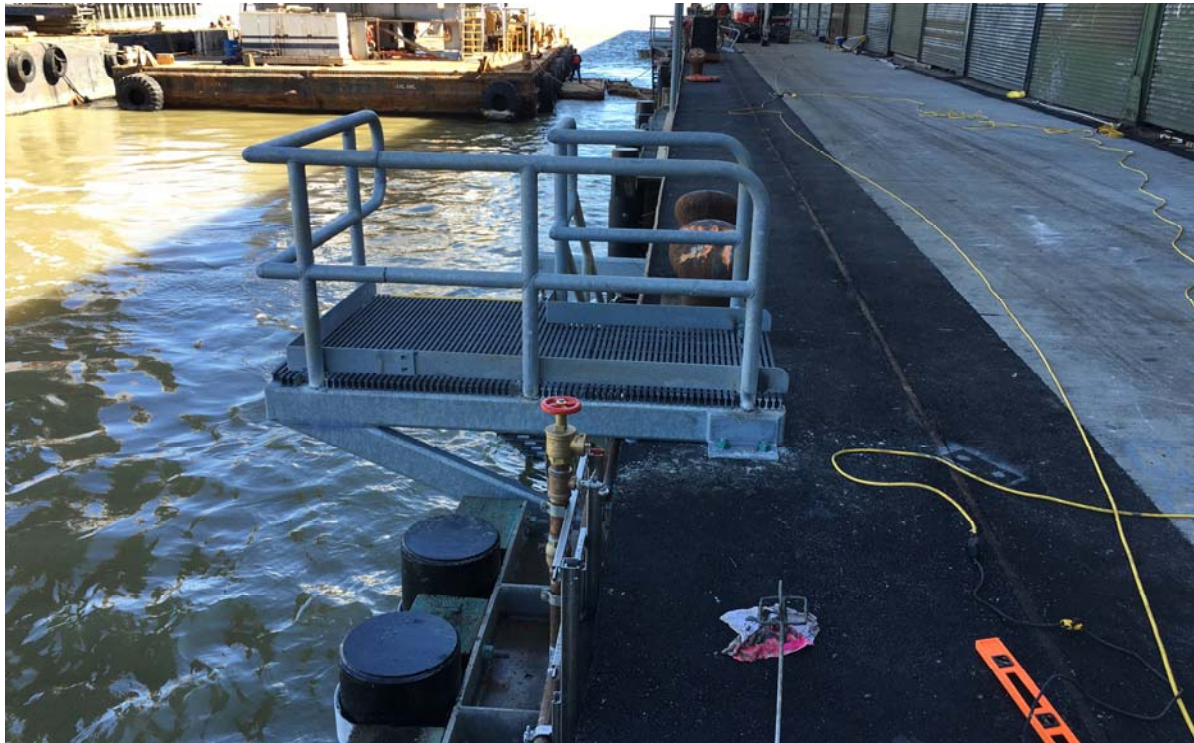
Pier 26 Fire Boat Berths – under construction
