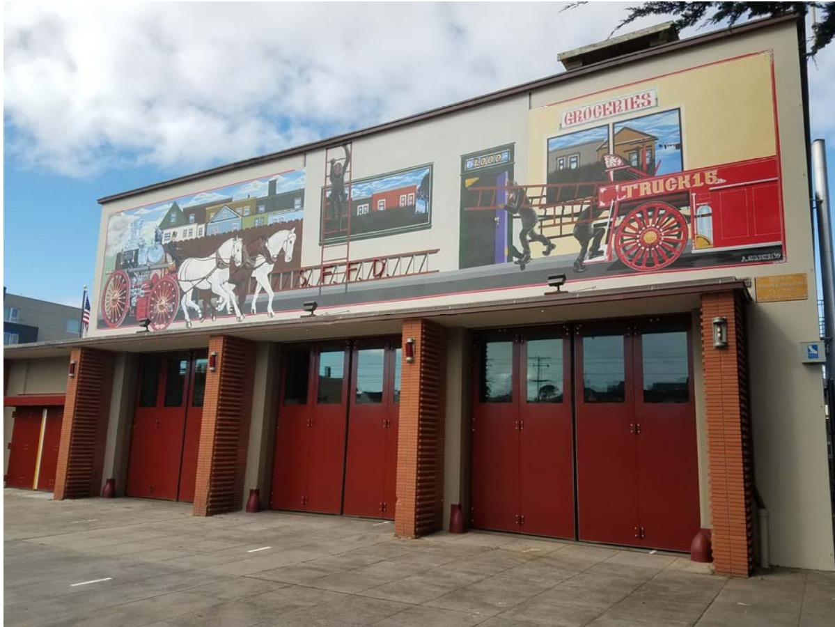
FS 15 Apparatus Bay Door Replacement – complete
