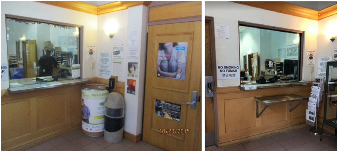
Richmond Police Station – Left: existing public transaction window with no accessible counter. Right: new public transaction window with accessible counter.
