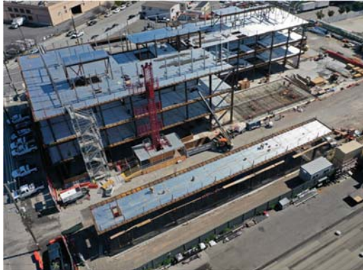
TCFSD – Structural Steel Erection (March 27, 2020)
