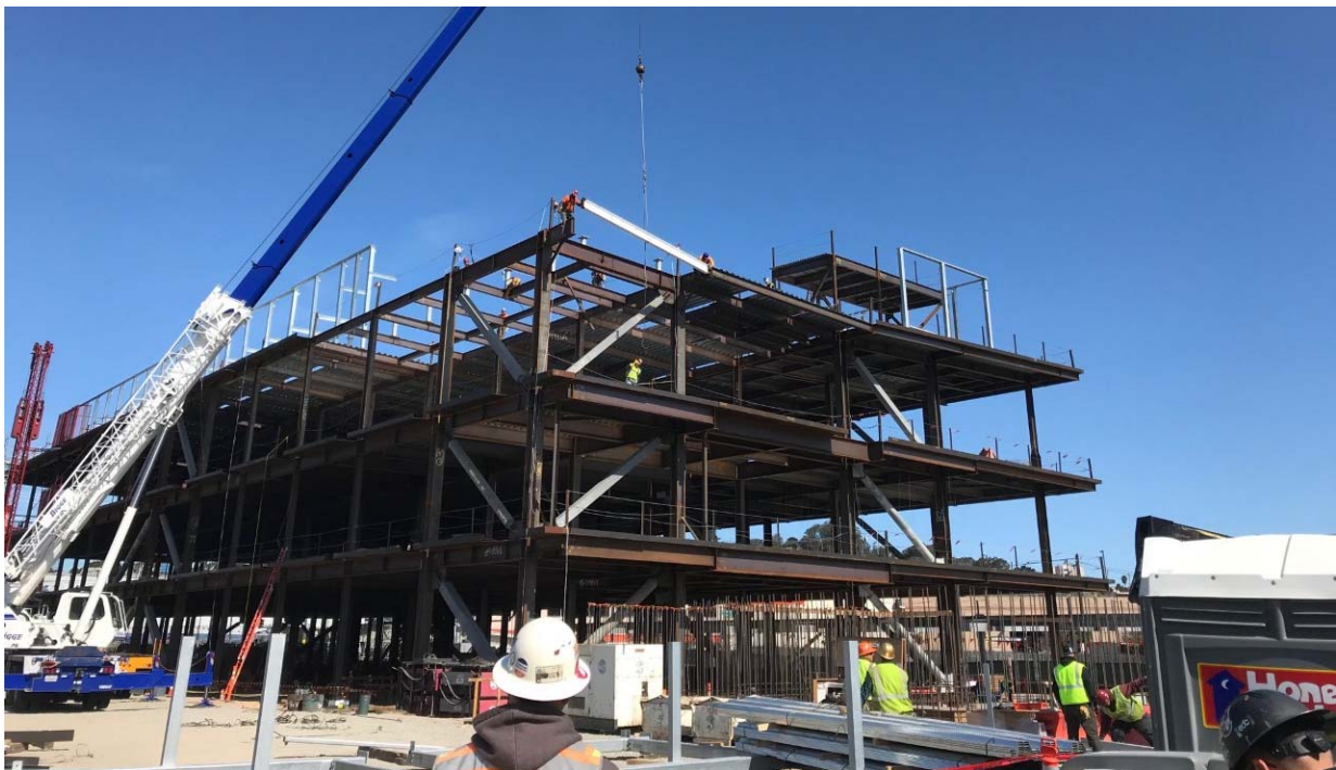
Structural Steel Topping Out Ceremony – April 3, 2020
