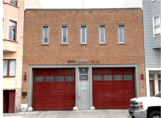
FS 28 – New Apparatus Bay Doors Installed (February 13, 2020)
