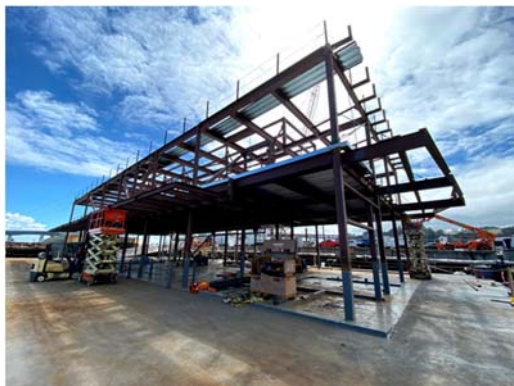
FS 35 – Structural Steel Complete (March 31, 2020)
