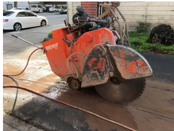
Richmond Station – sawcut existing asphalt for excavation and storm drainage installation
