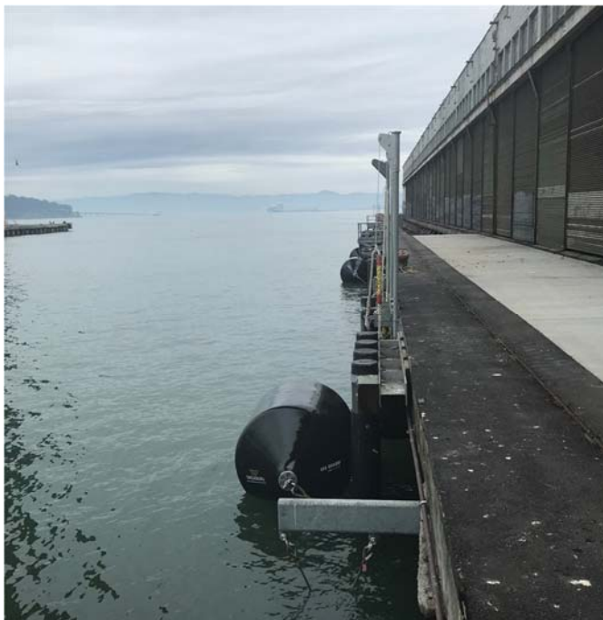
Pier 26 Fire Boat Berths – Fenders Installed (November 17, 2017)
