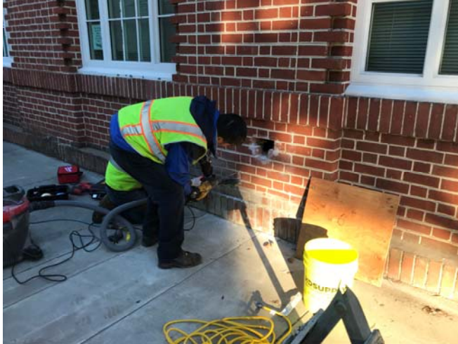
Richmond Station – brick removal to expose concealed downspout
