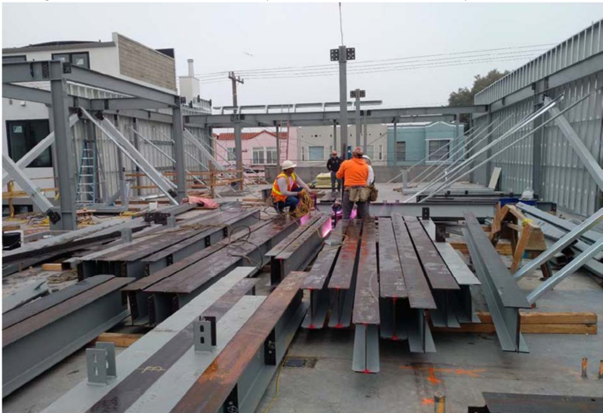
Fire Station 16 – Assembling Steel Members 2 nd Floor (December 27, 2017)
