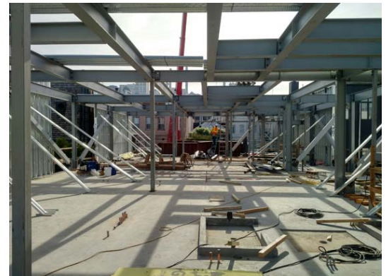
Structural Steel Framing at 2nd Floor (12/29/17)
