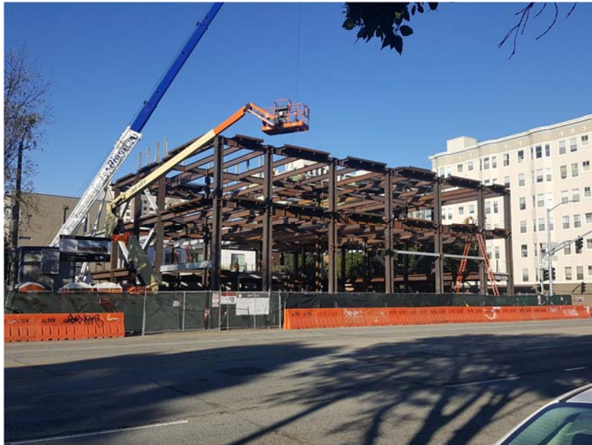
Fire Station 5 – View of Project Site from Webster Street (12/26/17)
