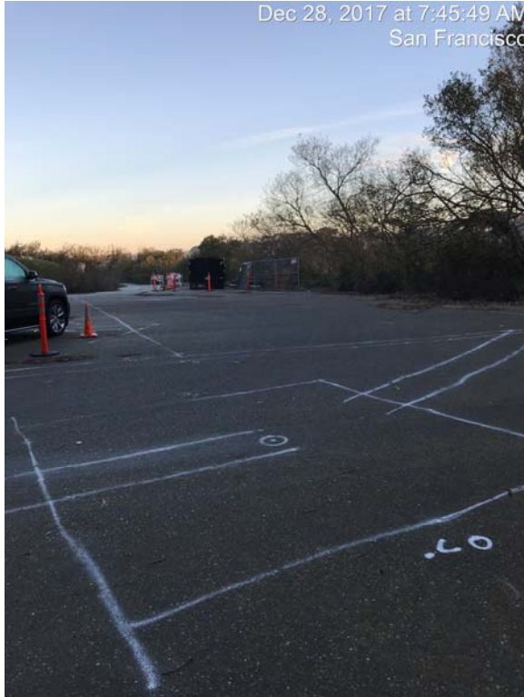
Lay-out for sump pump
