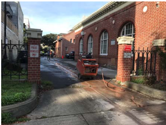
Richmond Station – sawcut existing asphalt for excavation and storm drainage installation
