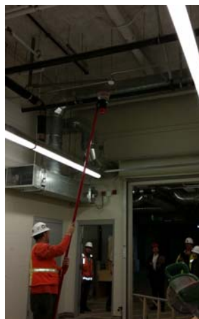
Fire alarm system testing
