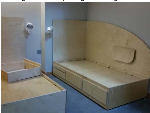
Installation of firefighter dormitory beds at FS4
