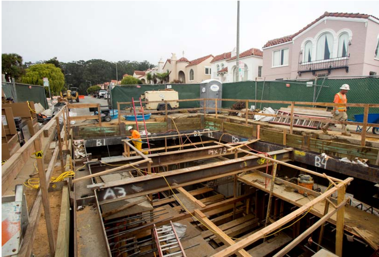
New cistern at 21 st Avenue and Ocean Avenue, October 2014
