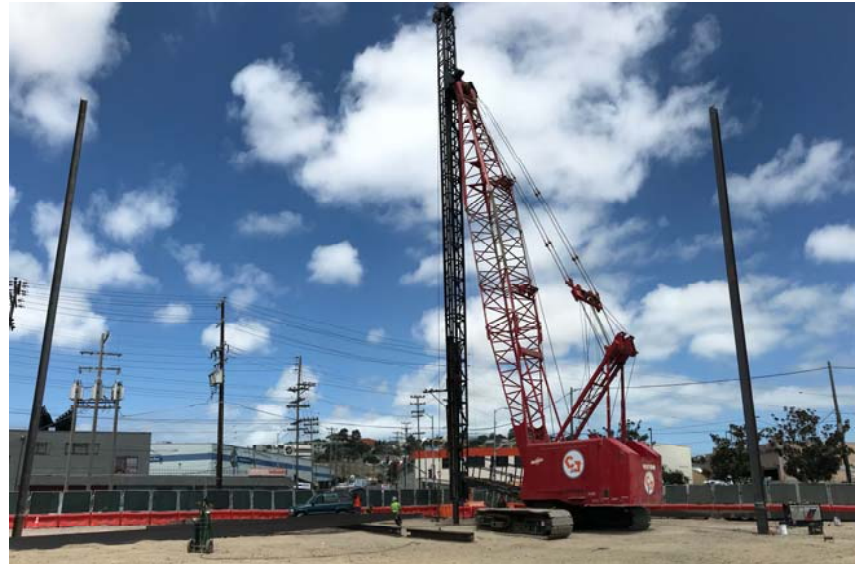
Traffic Company & Forensic Services Division Indicator Pile Program
