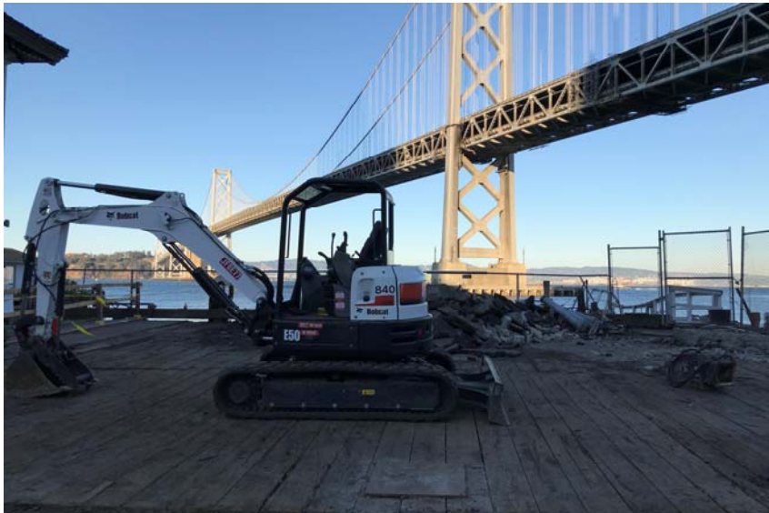
Fireboat Station No. 35 at Pier 22 1/2 Demolition of Asphalt Parking Lot
