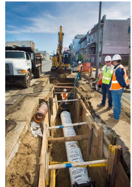
Irving Street Pipeline Project
