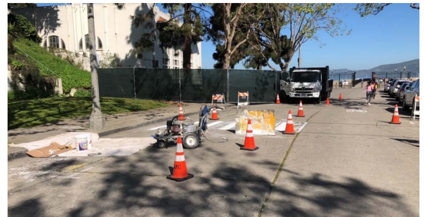
Pump Station 2 Project
