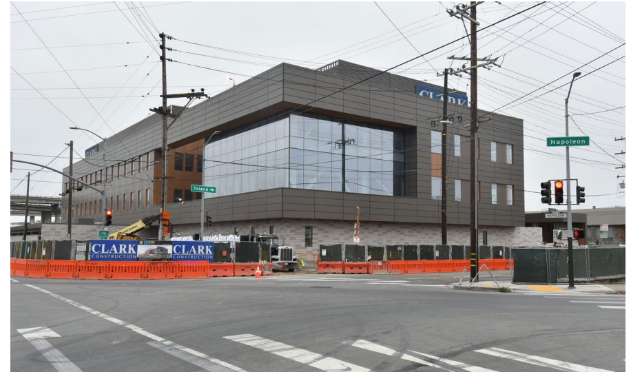
Traffic Company & Forensic Services Division Construction Progress at 1995 Evans Avenue
