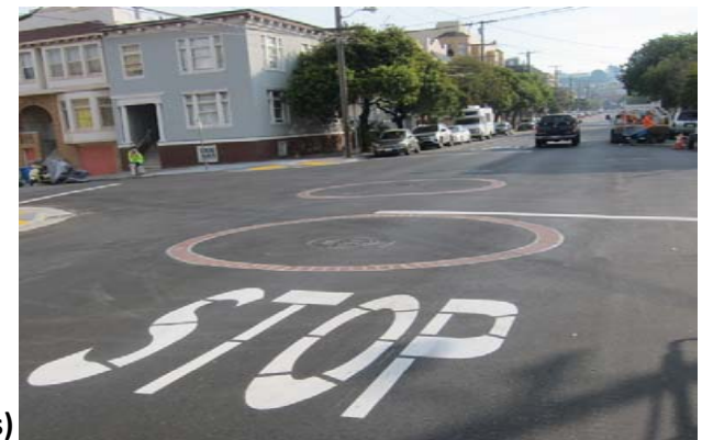
Cisterns (brick circles)
