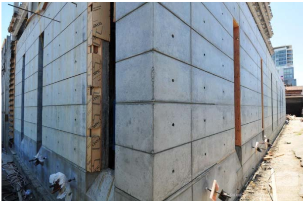
Architectural Concrete at 3 rd and Mission Rock St.
