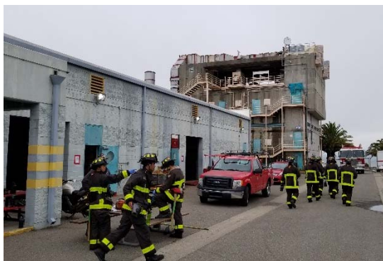
Existing SFFD Training Facility at Treasure Island
