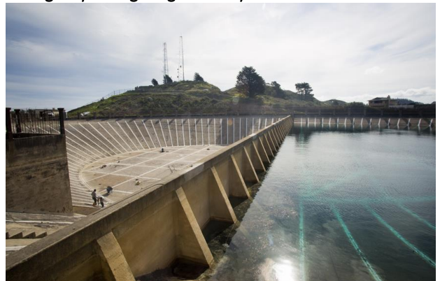
Twin Peaks Reservoir joint sealant
