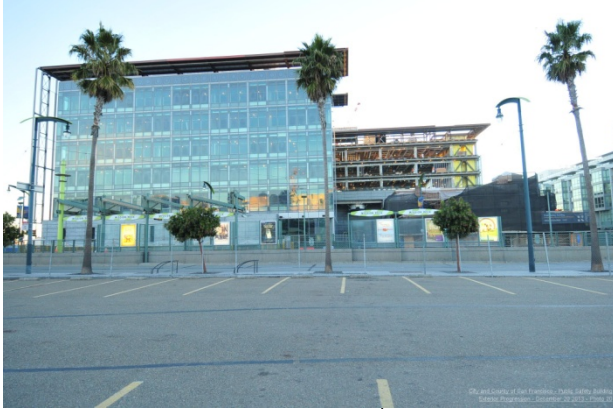
Exterior View of building from 3 rd Street
