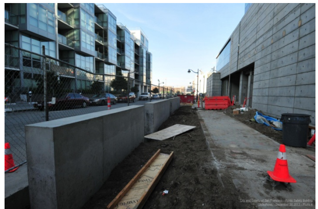
Anti-ram walls at China Basin St.
