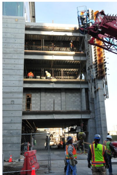
Conc. formwork removal
