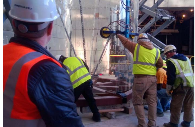
Installation of Police HQ Art
