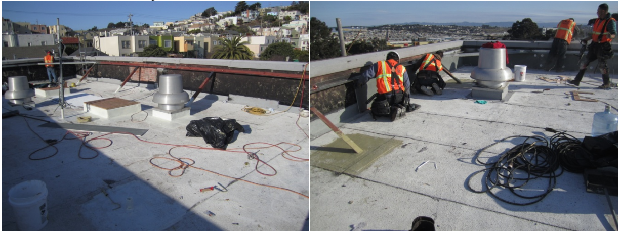
7438A Station 44 Roof Replacement
