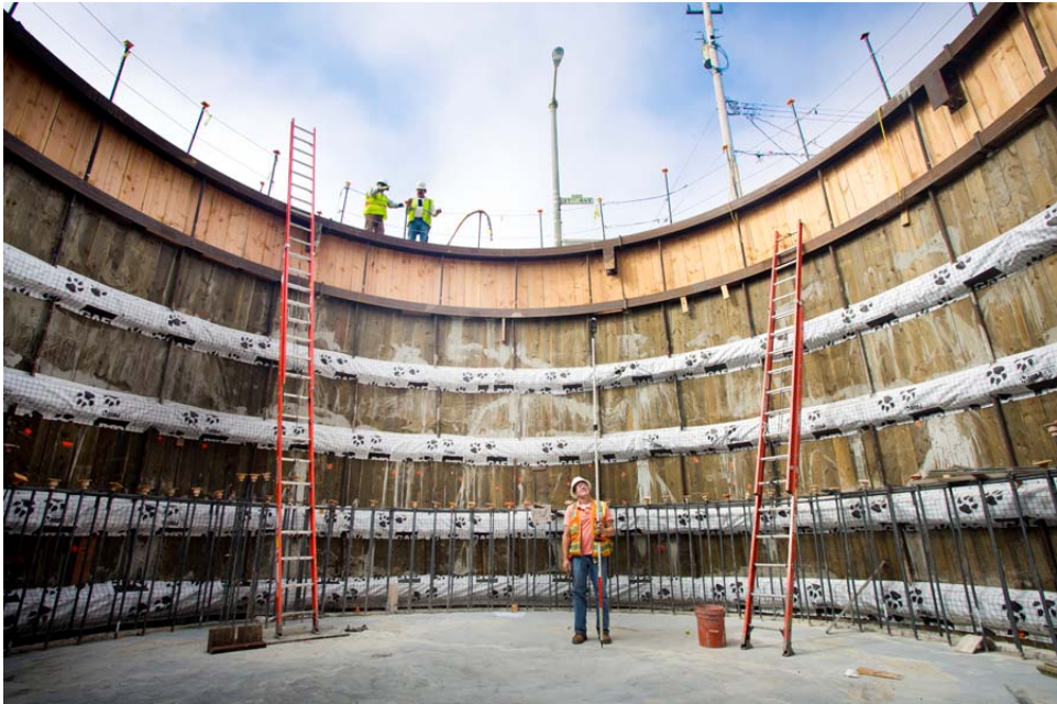
Confirming cistern floor slab elevation
