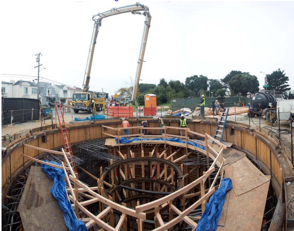
Placing cistern wall concrete
