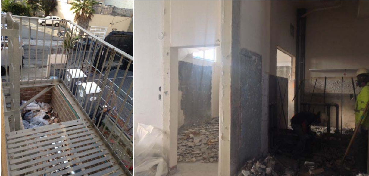
7427A Station 36 Selective Demolition
