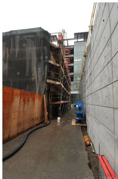
Walkway between FS30 and PSB
