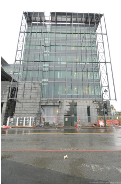
North façade screen framing
