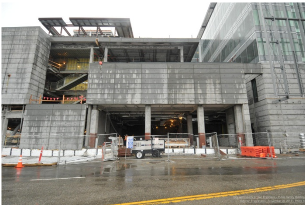
North Façade at FS4 Apparatus Bay
