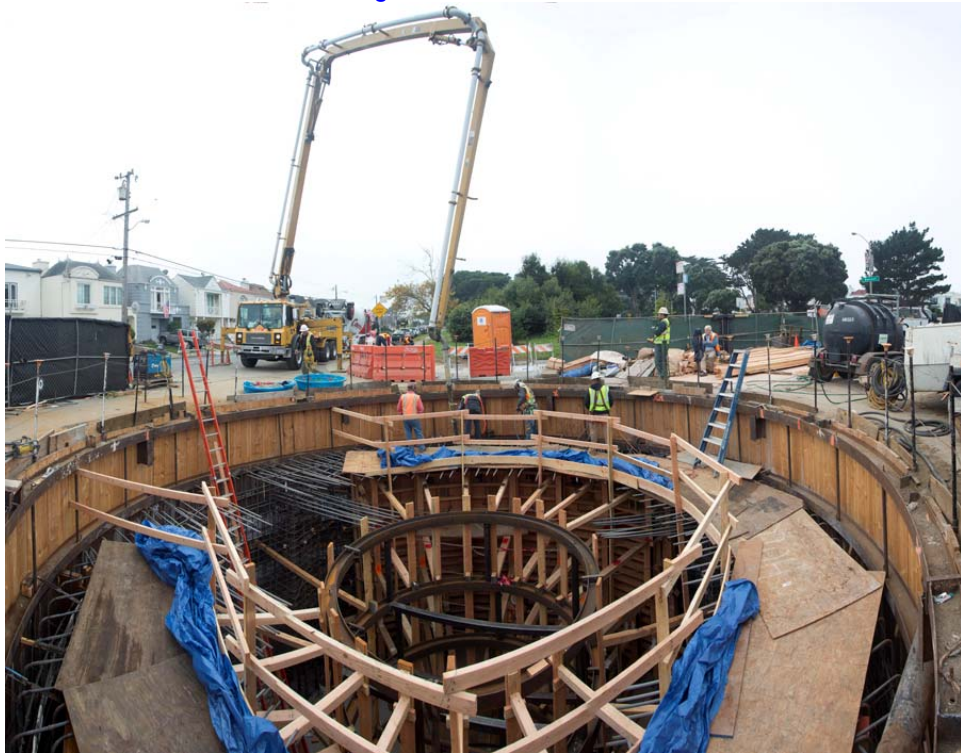
Placing cistern wall concrete
