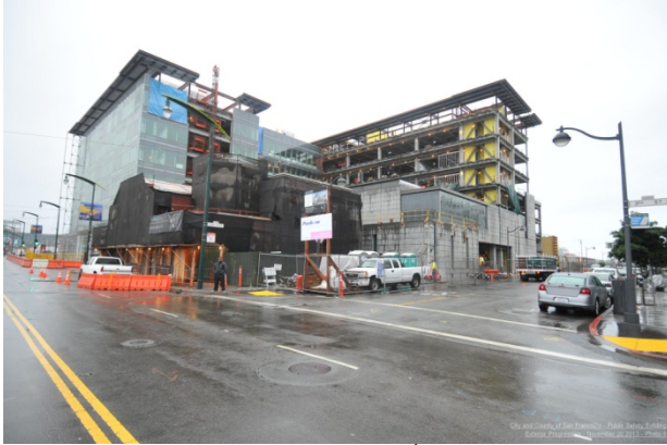
Exterior View of building from 3 rd Street
