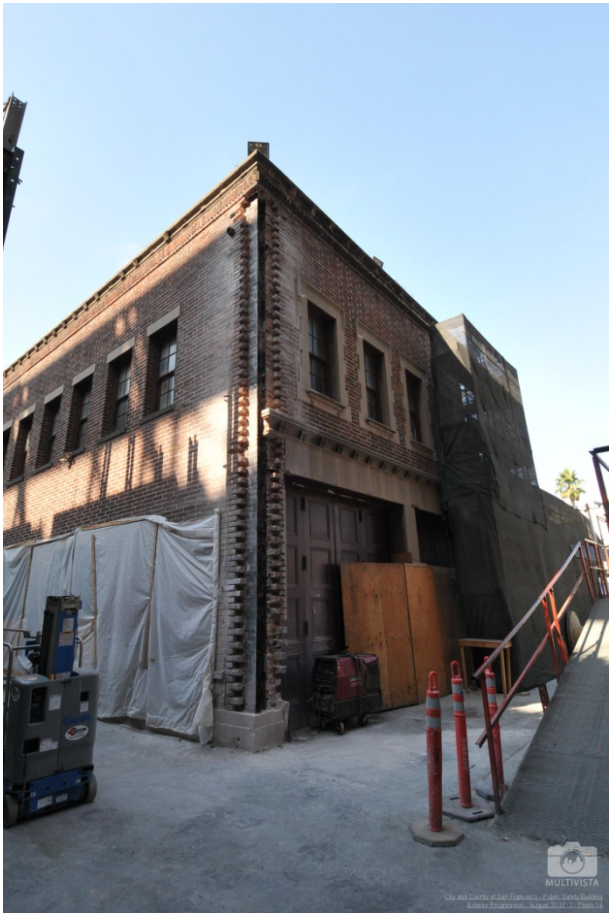
Fire Station 30 Structure - view of existing apparatus doors
