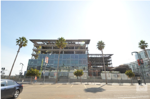
West Elevation of building (along 3 rd Street)
