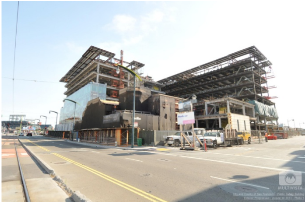
Exterior View of building from 3 rd Street (August 20)
