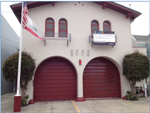
Exterior Envelope Station 40 Painting
