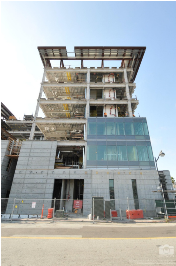
North façade of West Tower (from Mission Rock St.)
