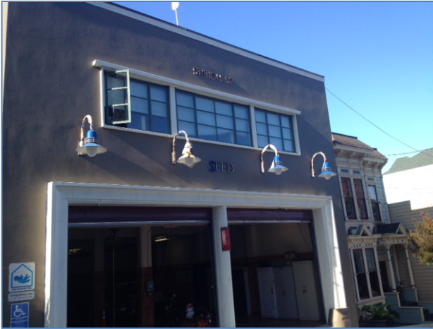
Exterior Envelope Station 32 Painting
