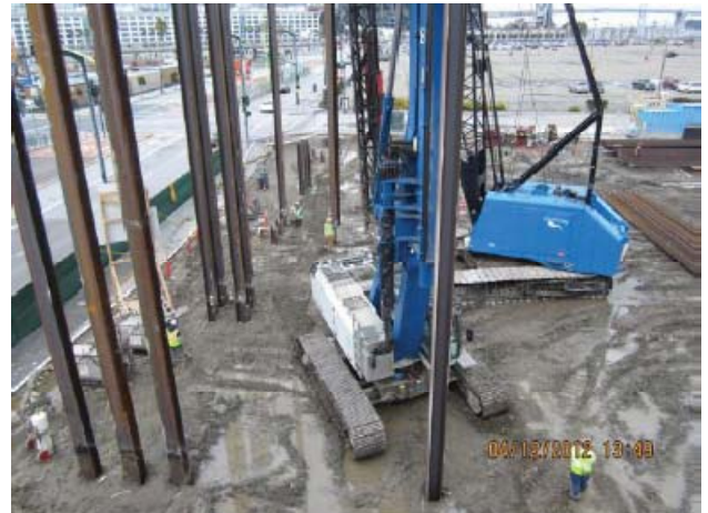
Installation of level 1 production piles
