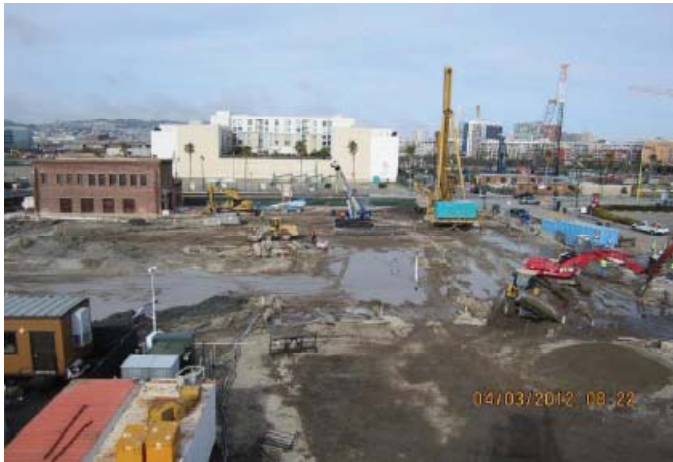
Project Site looking west towards 3 rd Street
