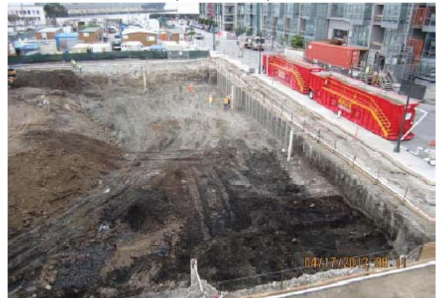
Lift #1 mass excavation in progress
