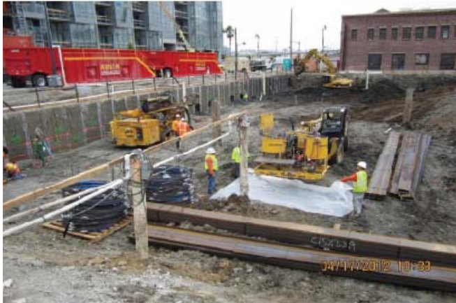
Tieback operation and mobilization
