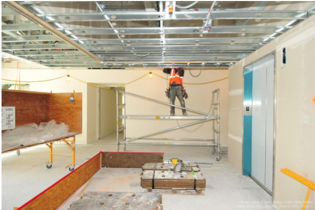
Ceiling framing at HQ visitor elevator lobby @ L3
