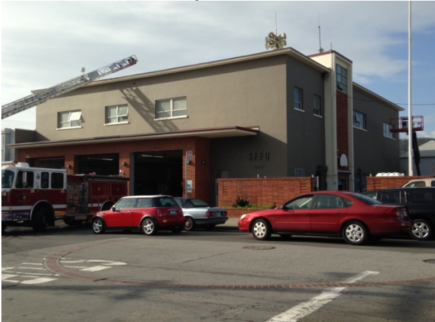
Station 17 Exterior Painting
