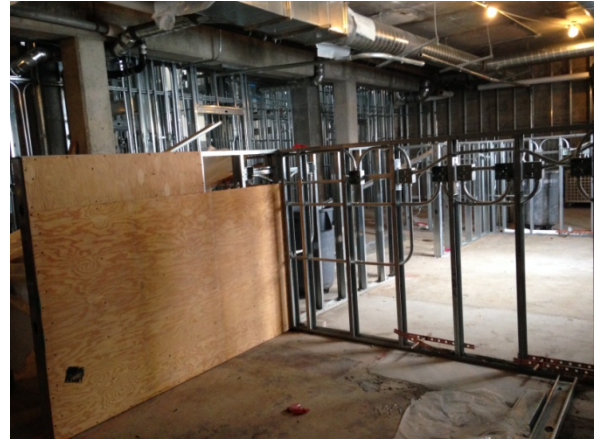
Framing at Second Floor
