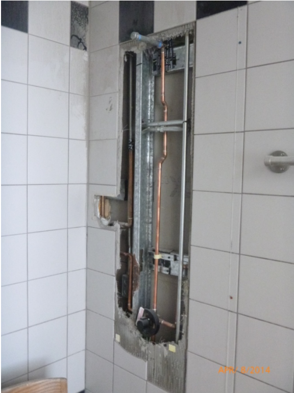
Rough Plumbing at Showers
