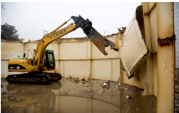
Ashbury Heights Tank Removal, March 2014
