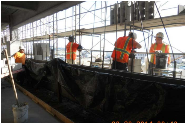
Installation of CMU wall at L4 parking
