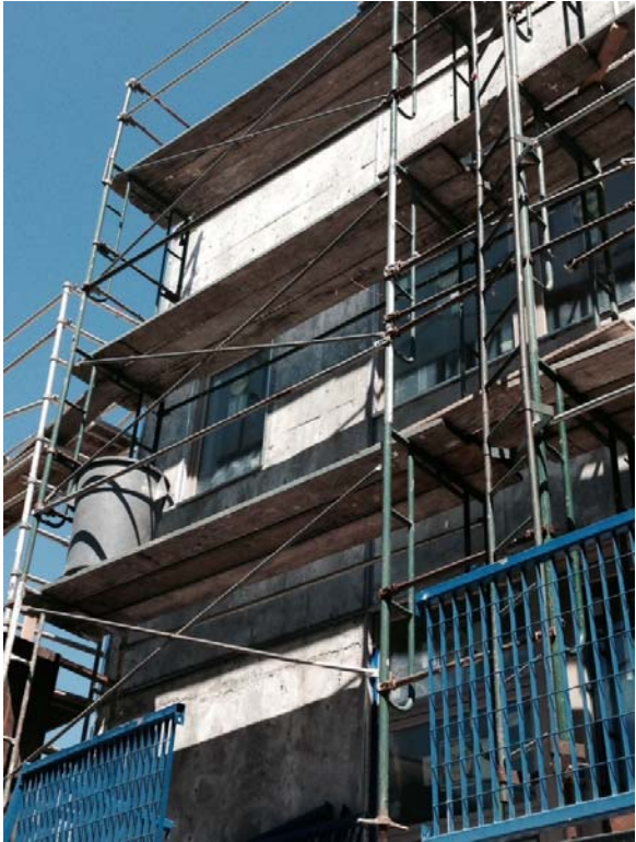
Ready for Stucco
