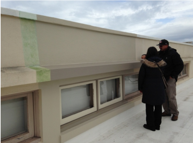
Station 18 Mock-up Review
