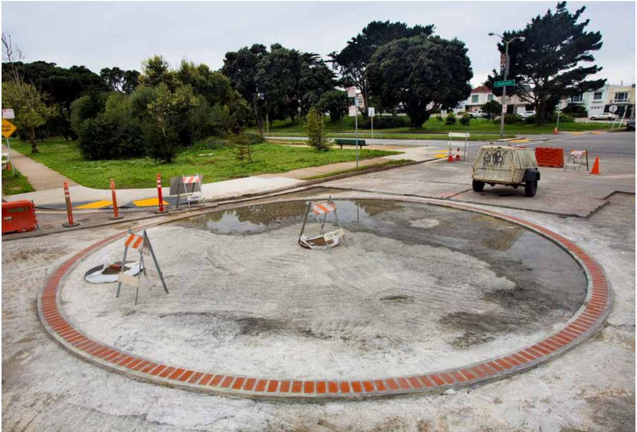
New cistern and Brick Ring, 36 th & Wawona, March 2014
