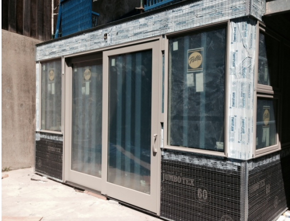
Ready for Stucco
