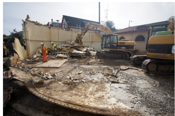
Ashbury Heights Tank Removal, March 2014
