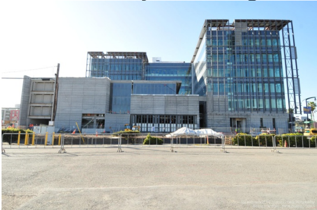
View of North Facade
