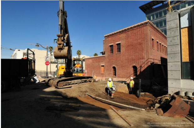
Site preparation at South Plaza
