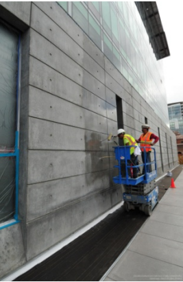
Application of anti-graffitti coating
