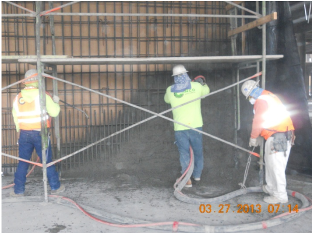
Shotcrete at Level 1 Wall.
