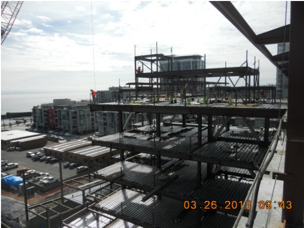
Structural Steel and Deck at Sequence 5.
