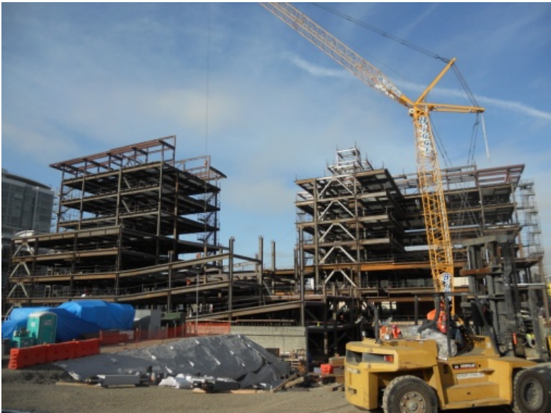
View of Building looking East.
