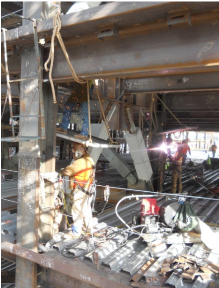
Welding at Level 3, Sequence 5
