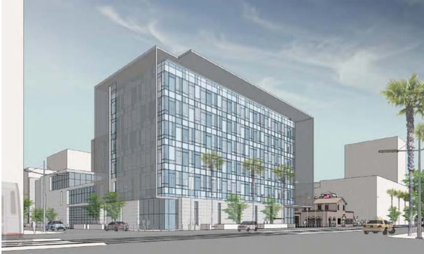
View from corner of Third Street and Mission Rock Street
