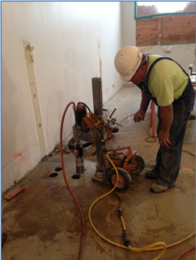
Slab Drilling for Vents
