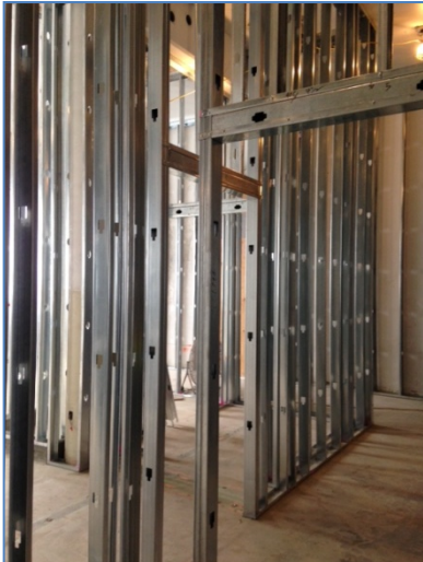
Metal Wall Framing
