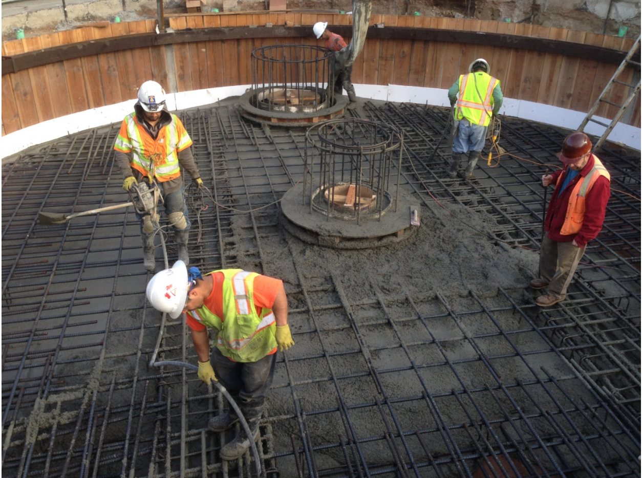
37 th Avenue/Lawton Street Roof of Cistern
