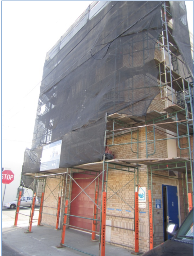
Exterior Preparation Work for Masonry
