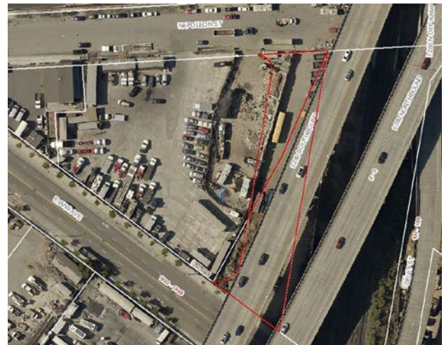
Public Works broke ground on a new Arborist Operations Yard at 1920 Evans Street (red parcel) that will house StreetTreeSF’s growing staff and fleet of vehicles.
