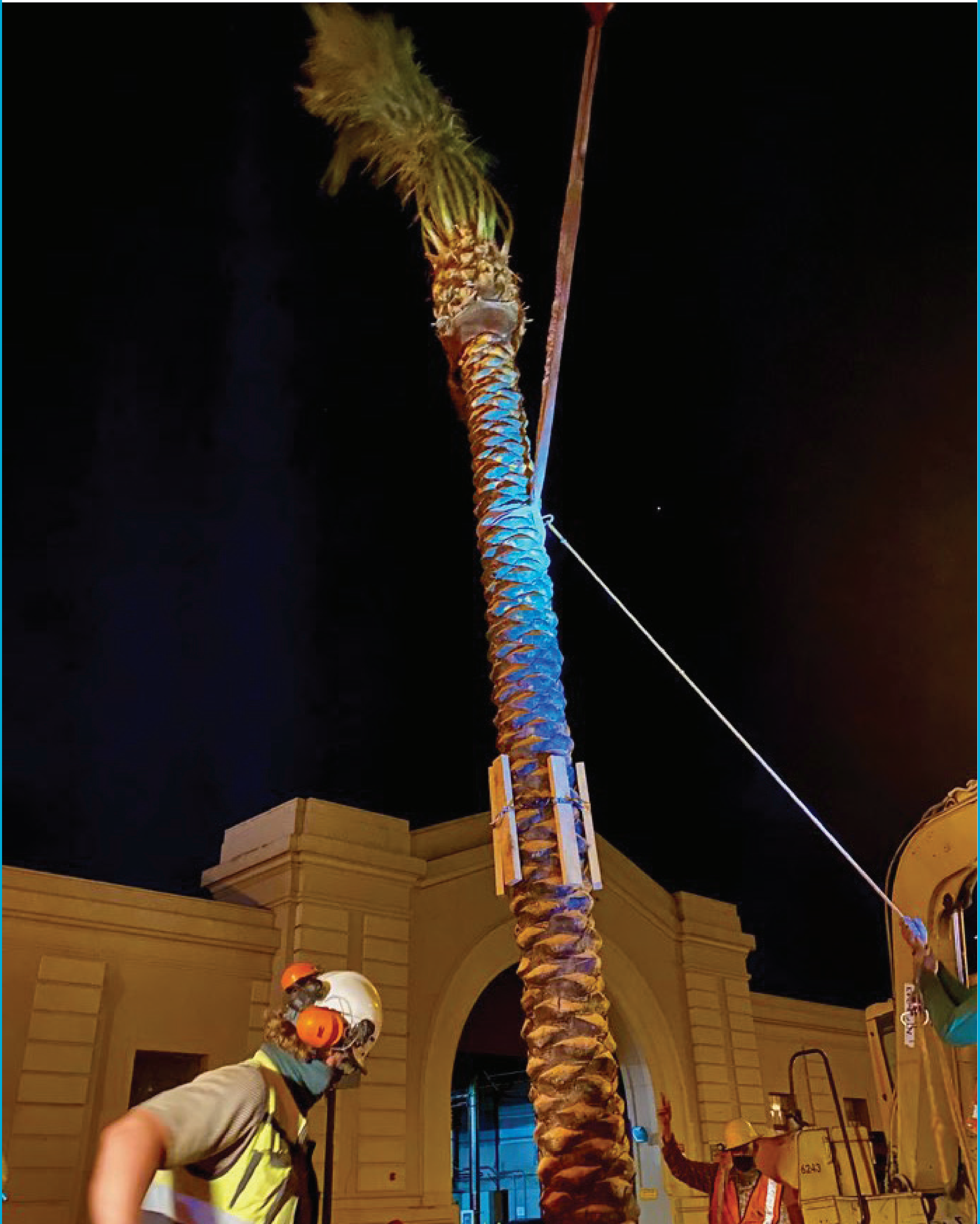
Crews used a crane to help place the towering palm tree in its new home on The Embarcadero.
