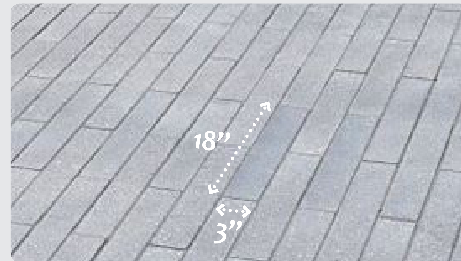
Linear Unit Pavers in Tree & Lighting Zone A
