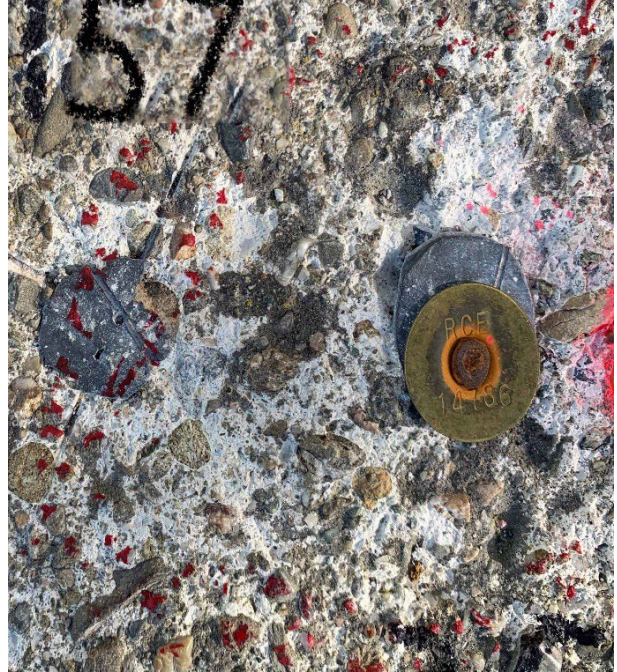
Nail and Brass Tag in Lead Plug
