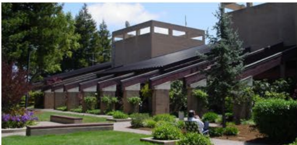
⑤ EXISTING ADMINISTRATION BUILDING
