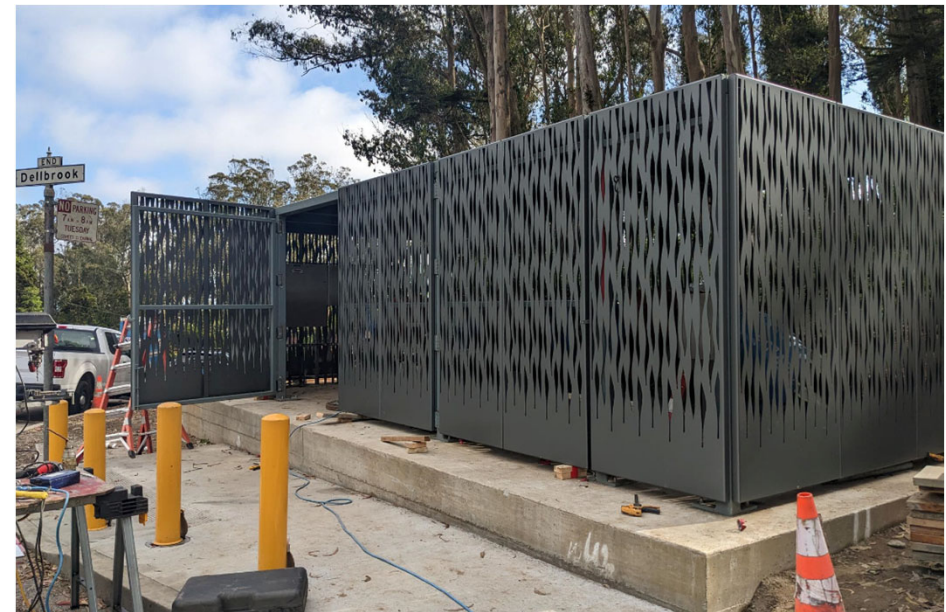
Clarendon Supply project: Enclosure installed
