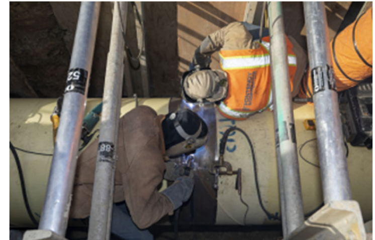
Installation of a new 36-inch (36") diameter welded steel pipe (WSP) at 19th Avenue and Sloat Boulevard
