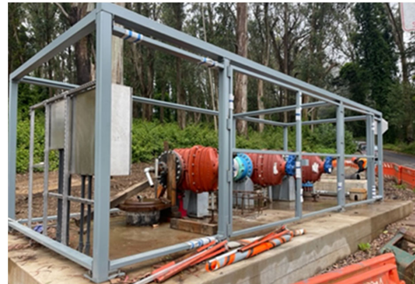
Clarendon Supply project: gate valve installation and enclosure
