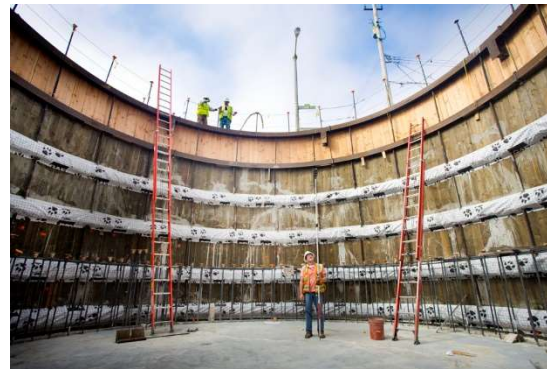
Construction of a Cistern, a Component of the EFWS
