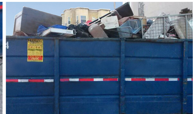
VIOLATION: No company name and exceeds allowable capacity
