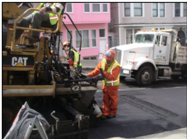
Crew Paving Street Block
