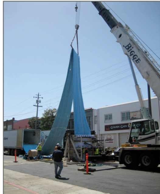
CIPP Liner Installation for an Existing 66" Concrete SD/Sewer Pipe
