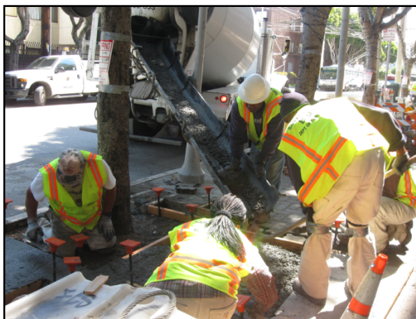
Staff Repairing Sidewalk in the Fillmore Jazz District
