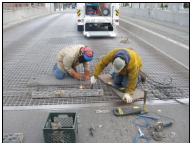
Staff Completing Maintenance Repairs on Islais Creek Bridge
