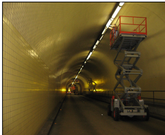
Crew Installing New Lights in the Broadway Tunnel
