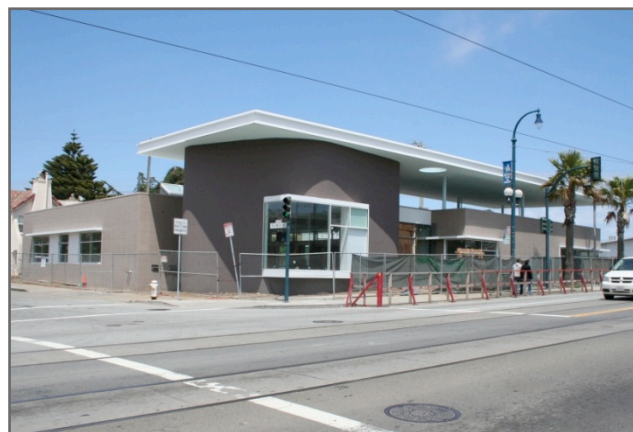
Ingleside Branch Library in Construction
