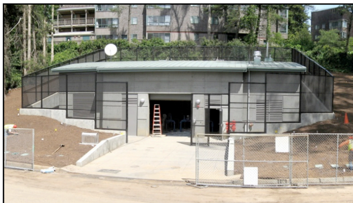
Forest Knolls Pump Station & Storage Tank
