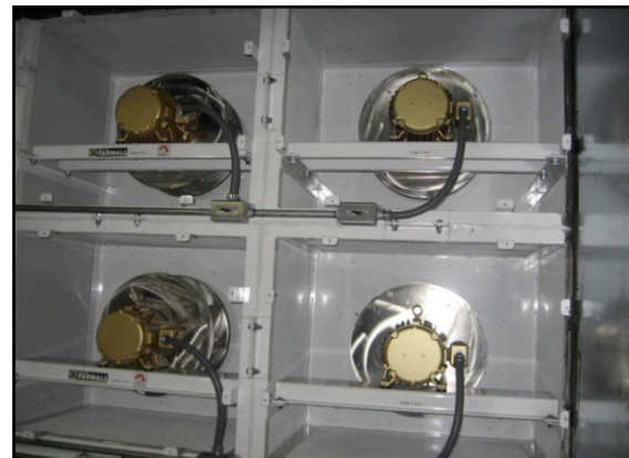
Installation of Modular Fan Wall Technology at the Hall of Justice
