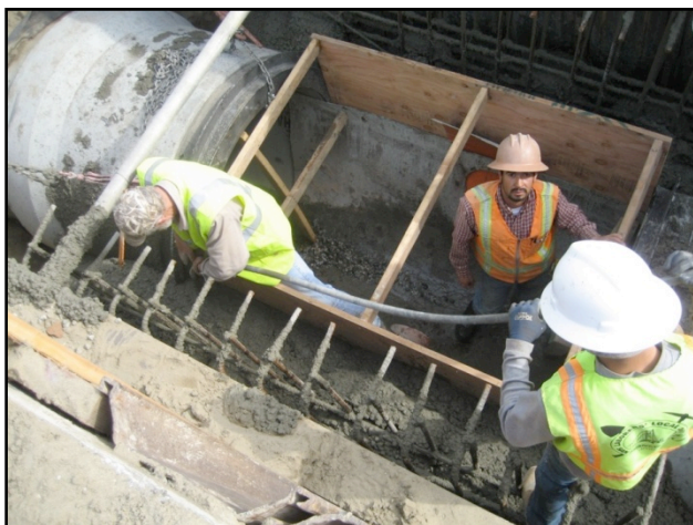
Sewer Pipe Replacement along Noriega Street
