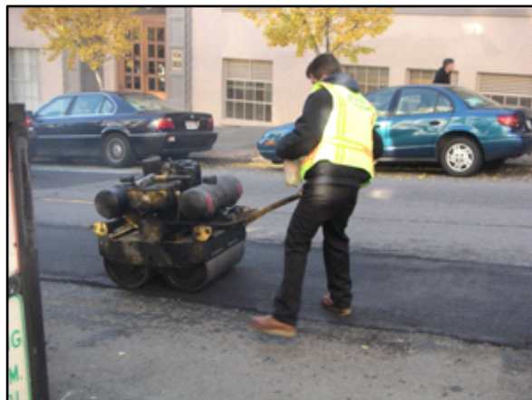
Staff Smoothing Out Asphalt on a Filled Pothole
