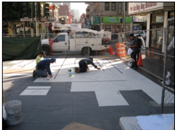
Construction crew installing artwork on the new art plaza on Broadway
