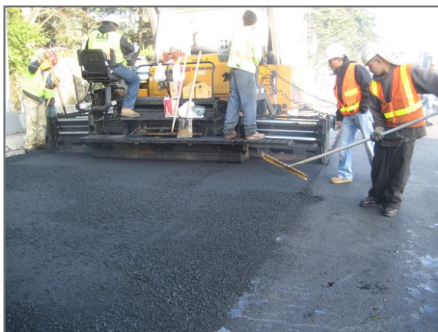
Contract Crew Repaving Street Blocks
