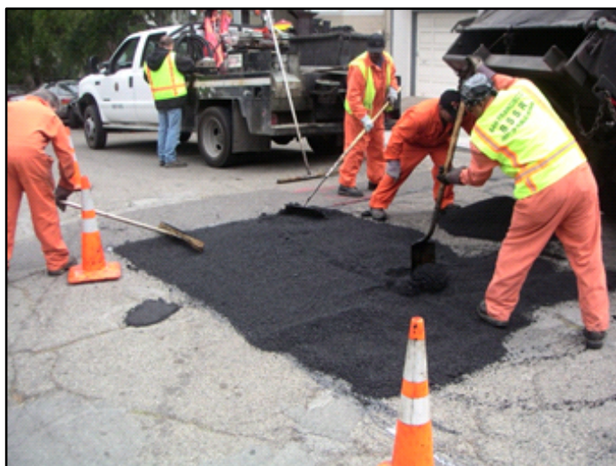
Crew Filling Pothole with Asphalt Produced by the City
