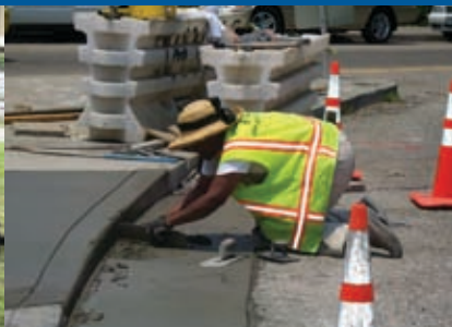
Cement work for new sidewalk and curb ramp
