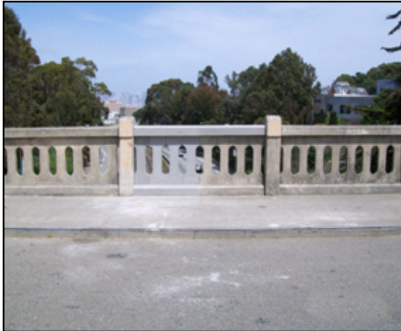
Repaired Highland Bridge
