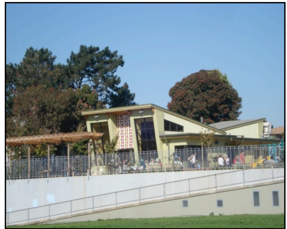
JP Murphy Playground & Clubhouse
