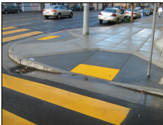
Newly constructed Curb Ramp for Safe Accessibility
