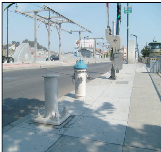
Relocation of a manifold at The Illinois Street Bridge
