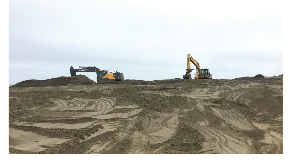
Public Works undertook the annual sand maintenance work along the Great Highway adjacent to Ocean Beach in June. The aim was to reduce the likelihood of sand buildup along the Great Highway during windy weather, forcing periodic closures of the roadway.
