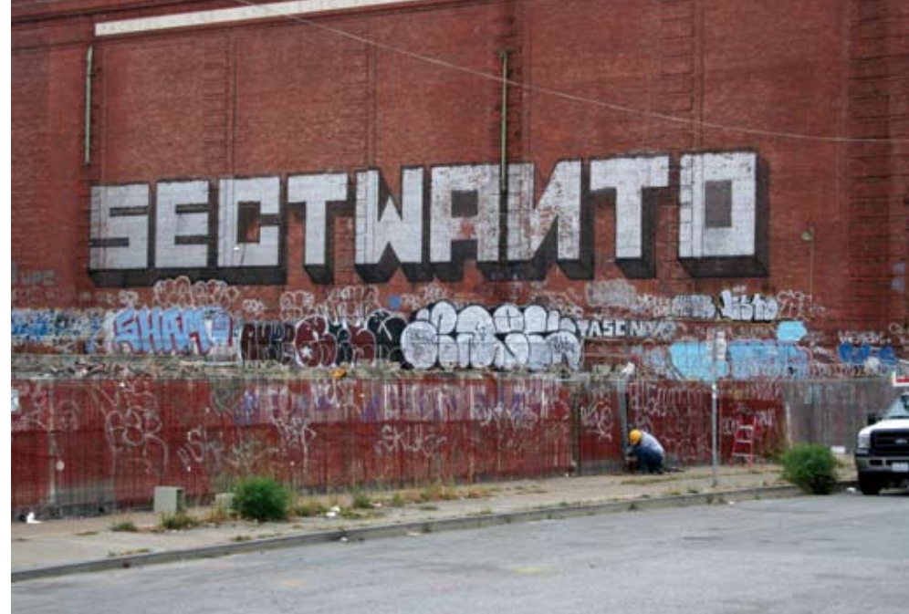
Mirant facility after abatement.
