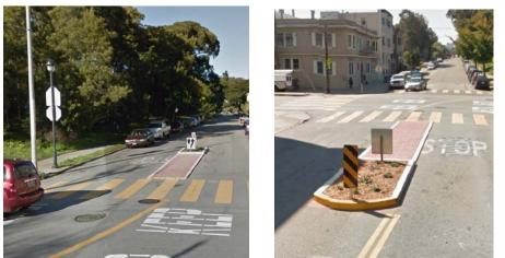
Raised island with mountable section for driveway and emergency vehicle access
