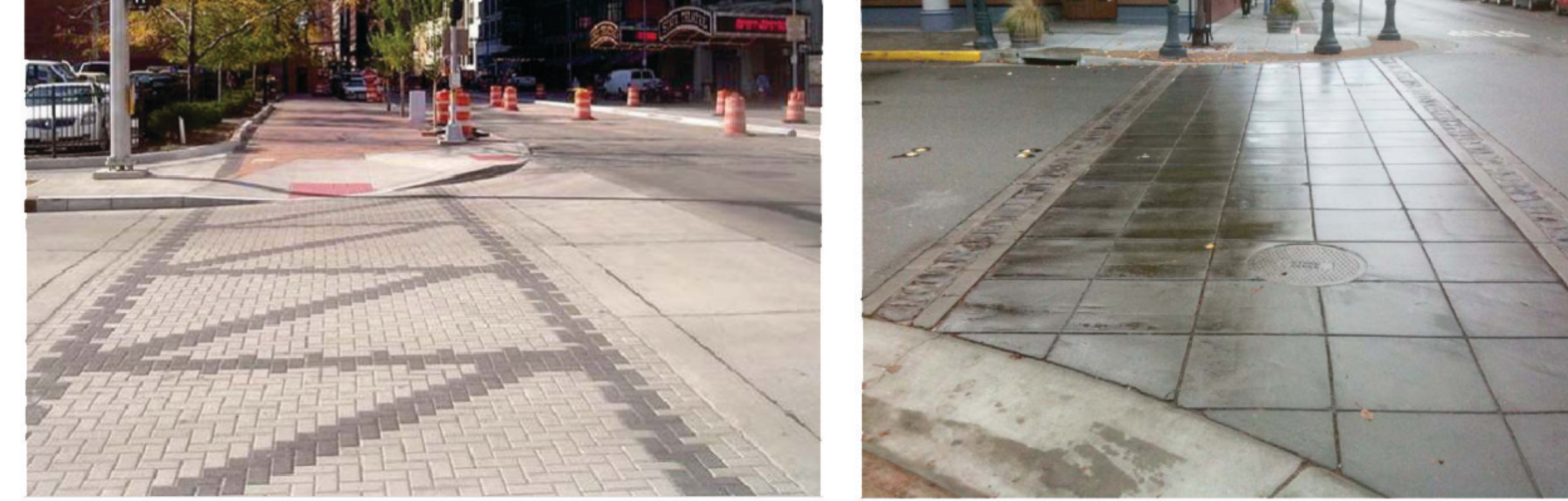
SPECIAL CROSSWALK PAVING
