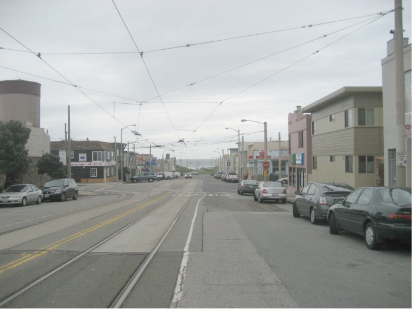
TARAVAL VIEW WEST FROM 46TH AVENUE
