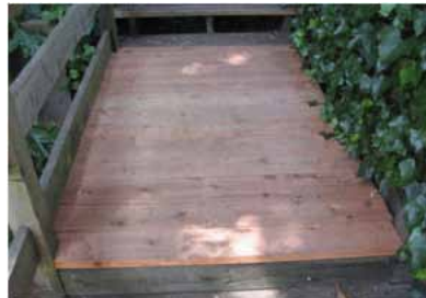
Filbert Street Stairway (before and after)
