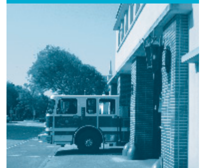
Neighborhood Fire Stations
