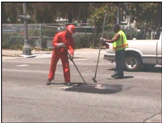
BSSR crew repairs pothole
