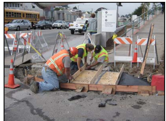
BUF crew repairs walkway
