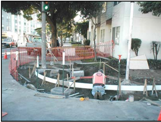
Installing Code Compliant Curb Ramps
