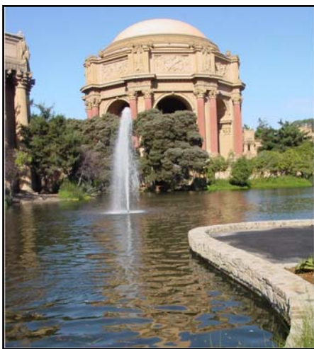
The lagoon edge with added stone wall is part of Phase I
