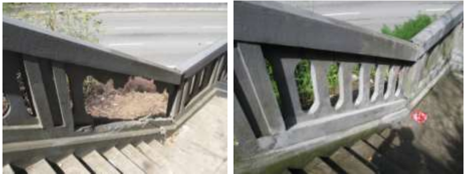
San Jose Avenue stairway – before and after
