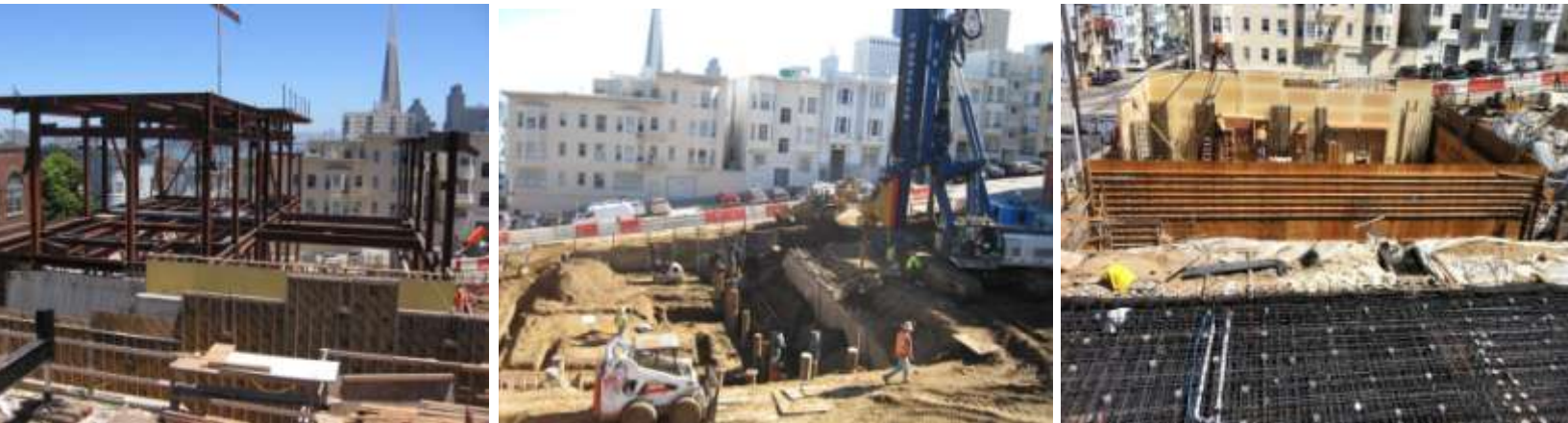
Chinese Recreation Center construction
