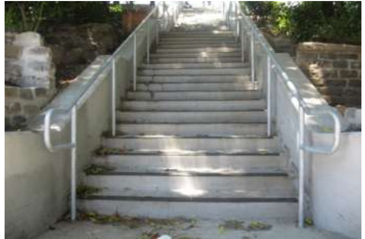
Before and After of Corbin Place Stairway Replacement
