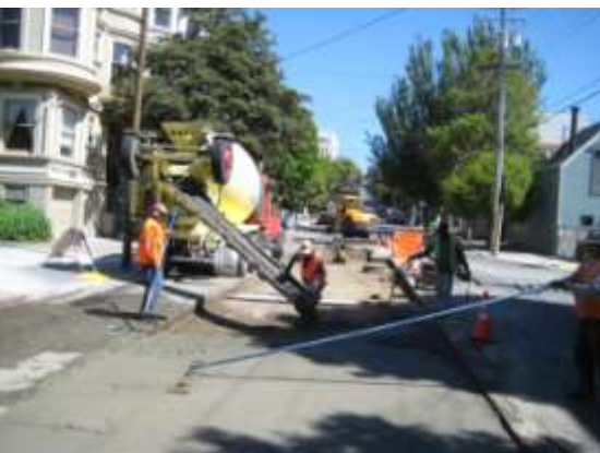
Waller, Sanchez and Steiner Streets Pavement Renovation
