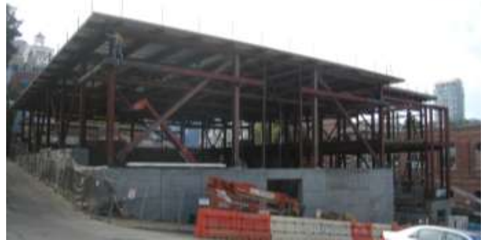
Chinese Recreation Center - Steel framing of gym
