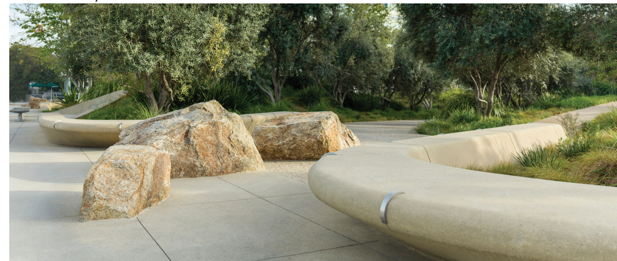
PRECAST CONCRETE WALL W/ BOULDERS
