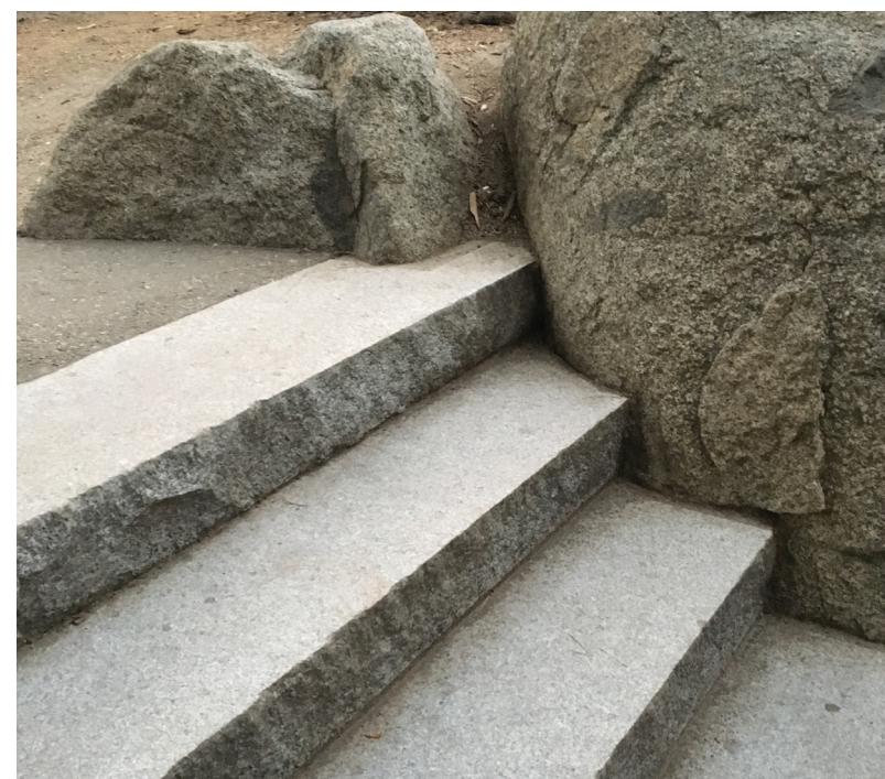
BOULDER CHEEK WALL DETAIL
