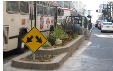
Market at Kearny Streets. The project replaced a concrete MUNI crash barrier with landscaped planter
