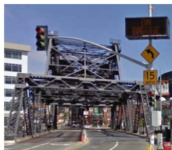
3 rd Street Bridge
